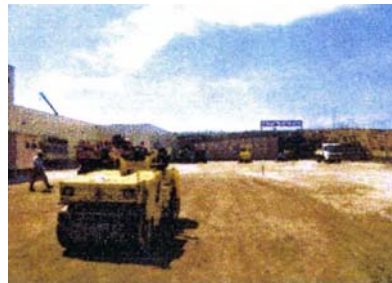
②路盤撤出・転圧
