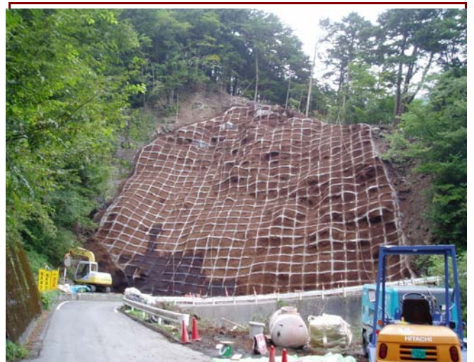
枠内植生基材吹付
